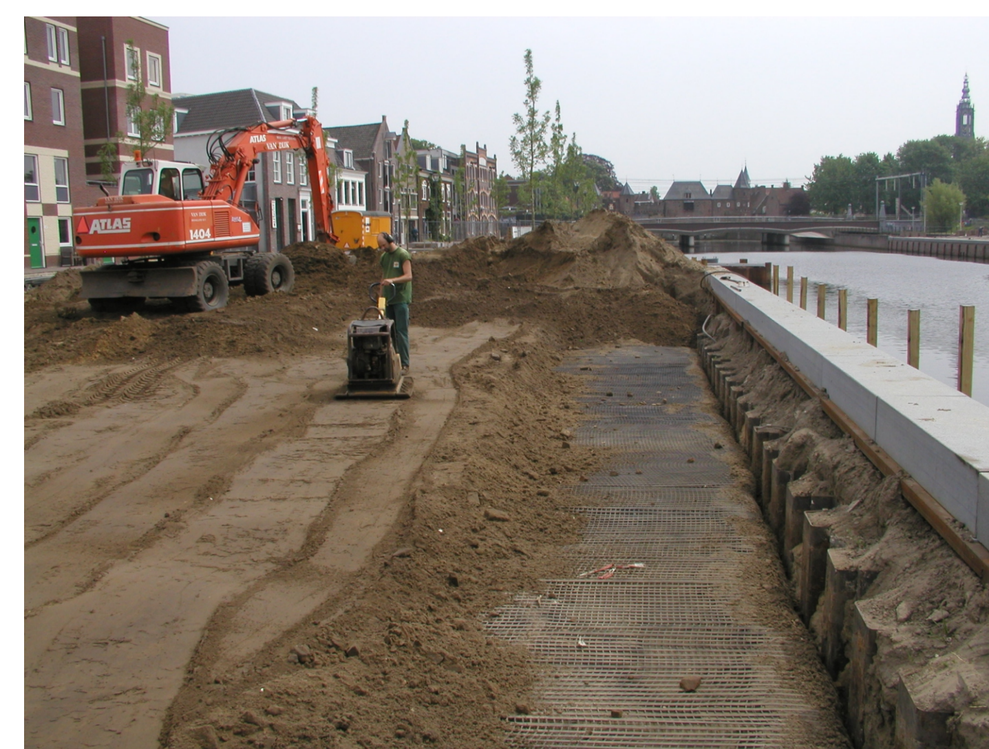
backfilling and compacting
