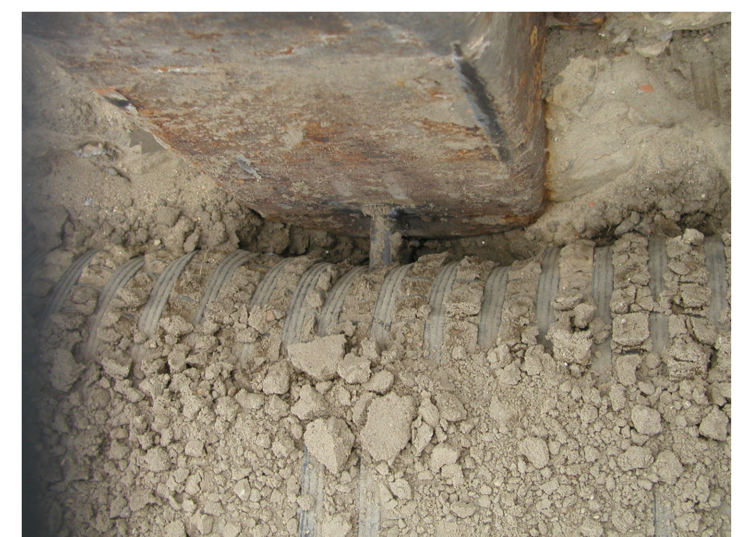
well tensioned geogrid after compaction
