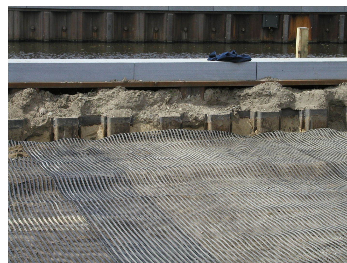
"slacky" placed geogrid
