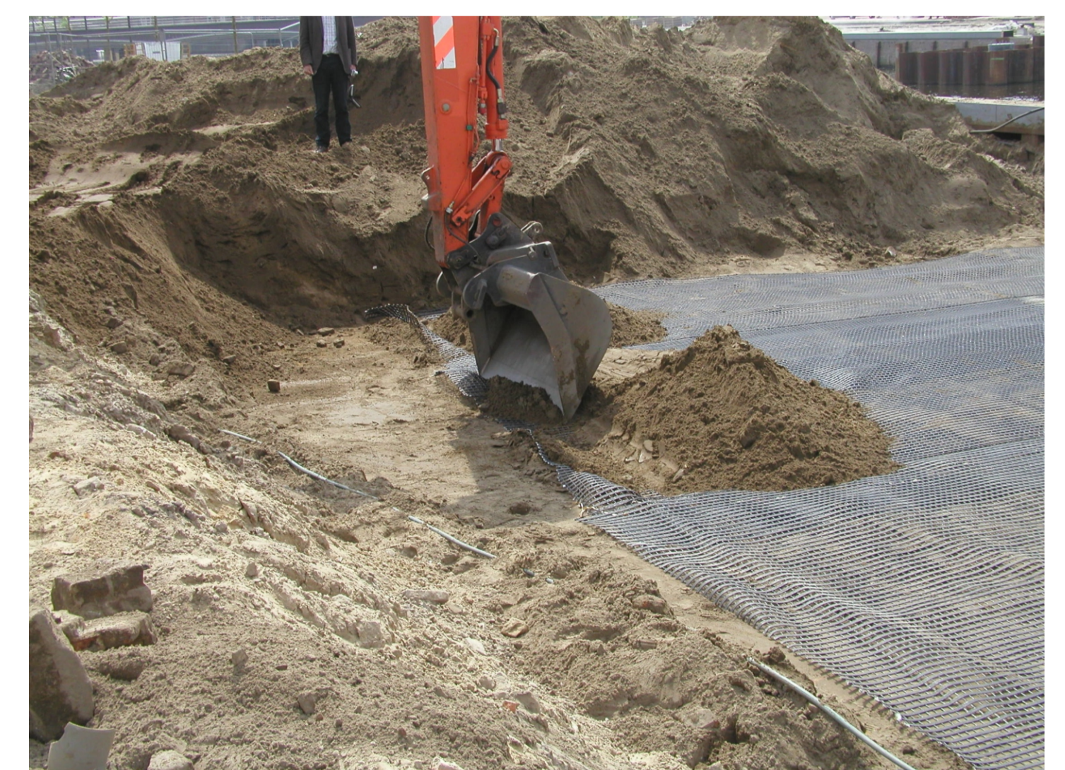
fixing & tensioning the geogrid with the excavator shovel
