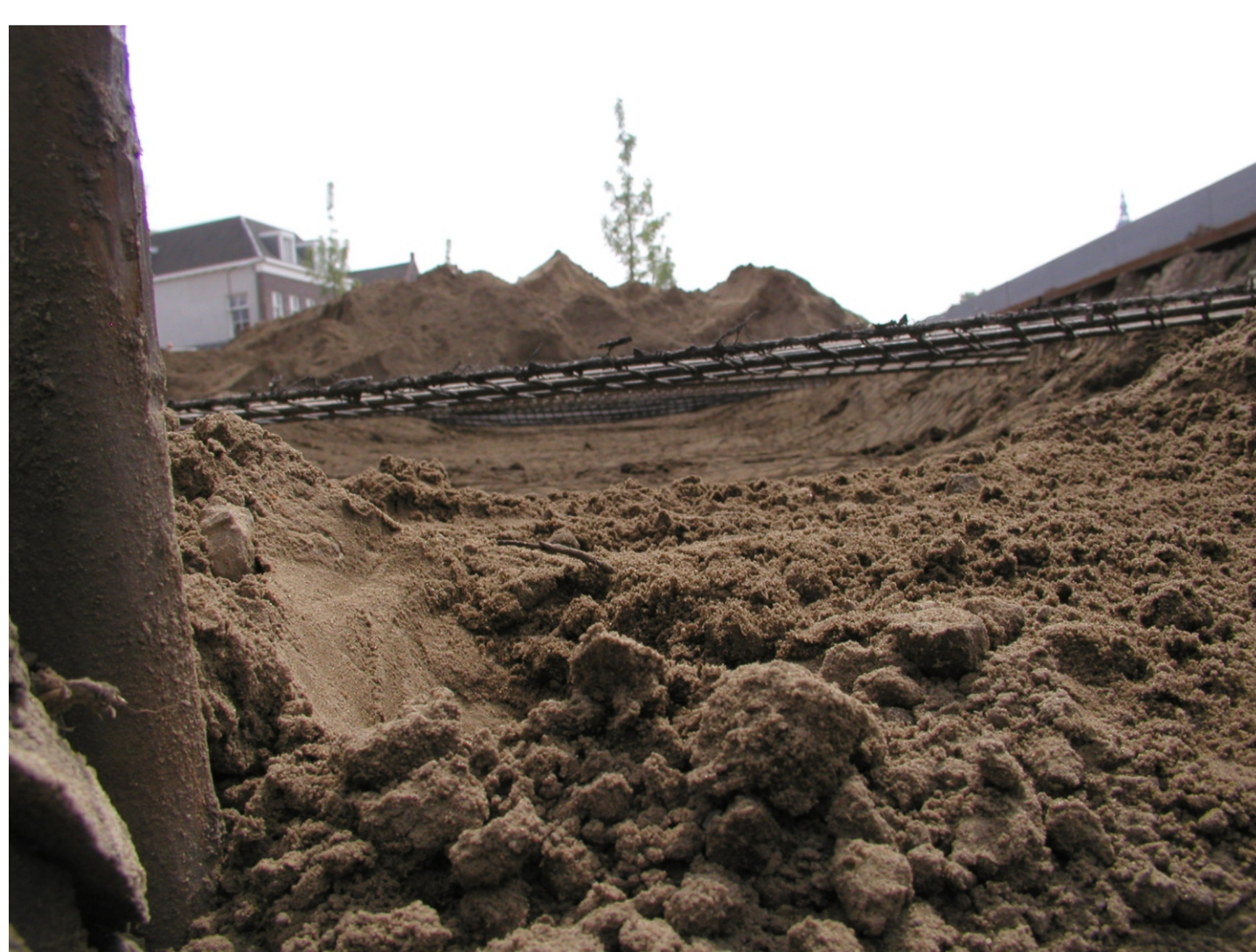
tensioned geogrid over the trench
