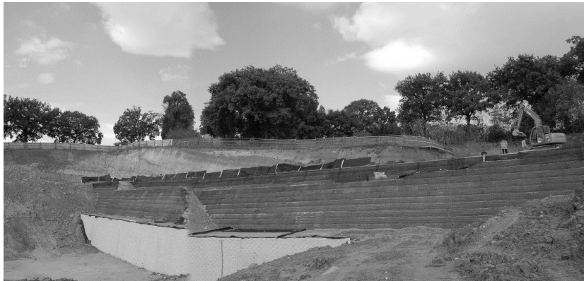
Figure 6. View of SRS during construction.
