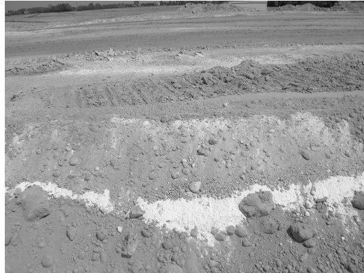
Figure 2. Lime stabilized soil.
