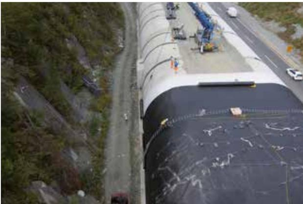
Installation of primary 2.0 mm PE-HD waterproof barrier, welded and leakage-tested.
