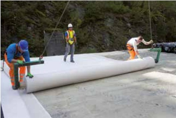
Installation of Tektoseal Clay 5000+ as self-healing, secondary waterproof barrier
