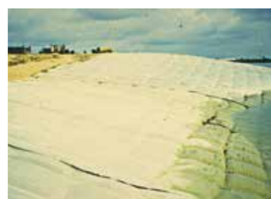
1983 Warri River Nigeria Deckwerk Incomat® Flex
