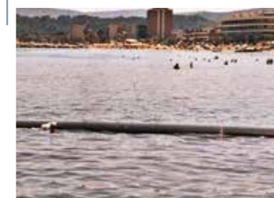
2002 Le Lavandou France Breakwaters SoilTain® Tubes
