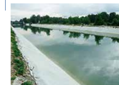
2013 Mittlere-Isar-Kanal Germany Canal refurbishment Incomat® Standard
