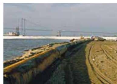
1986 Wilmington Harbour USA Land reclamation Stabilenka®
