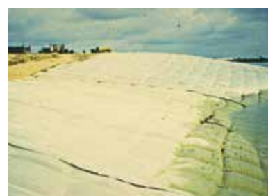
1983 Warri River Nigeria Revetment Incomat® Flex
