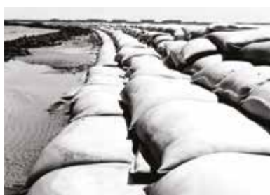
1963 Rüstersieler Watt Germany Dike construction SoilTain® Bags
