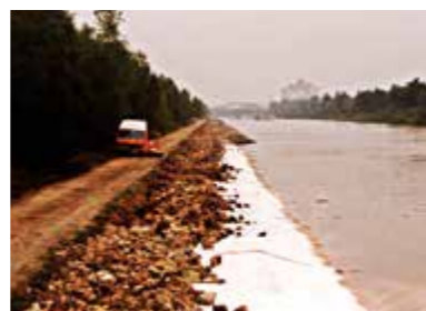
1989 Mittellandkanal Germany Revetment HaTe® Nonwovens
