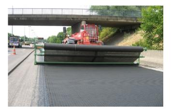
The unrolling can be undertaken with the help of a simple system, either manually, or mechanically when using wider, heavier rolls.
