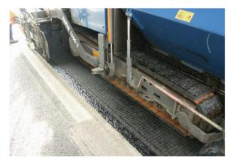
The reinforcement grid must be laid free of folds and waves. However, if a slight wave builds up in front of the paving machine, this will not detrimentally affect the performance of the reinforcement. Joints in the asphalt pavement must not coincide with overlaps in the rolls of reinforcement grid. The current technical requirements for the compaction of asphalt layers must be observed when using HaTelit.
