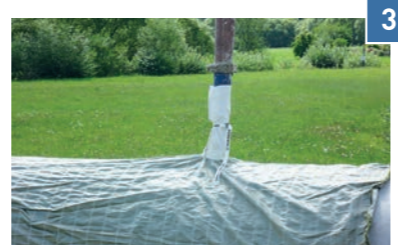
Concreting via filler neck
