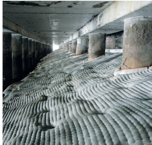
Bed protection Guatemala, 2016, slope and bed protection at new Quetzal port terminal using Incomat Standard.
