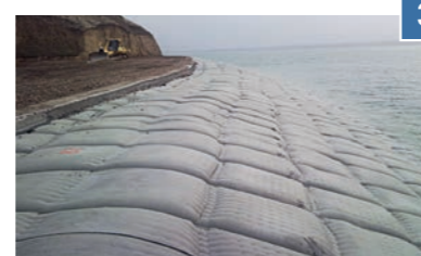
Filling of panels with fluid concrete/mortar
