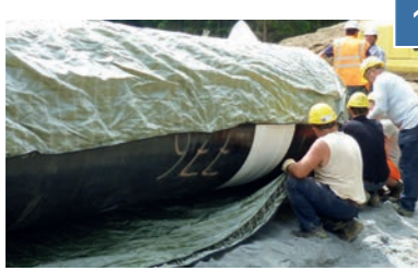
Fixing to pipe section
