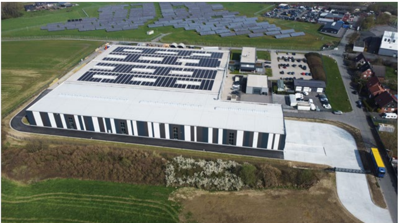
Aerial view of the expanded 'Im Brömken' production site, Credit: © GOLDBECK
