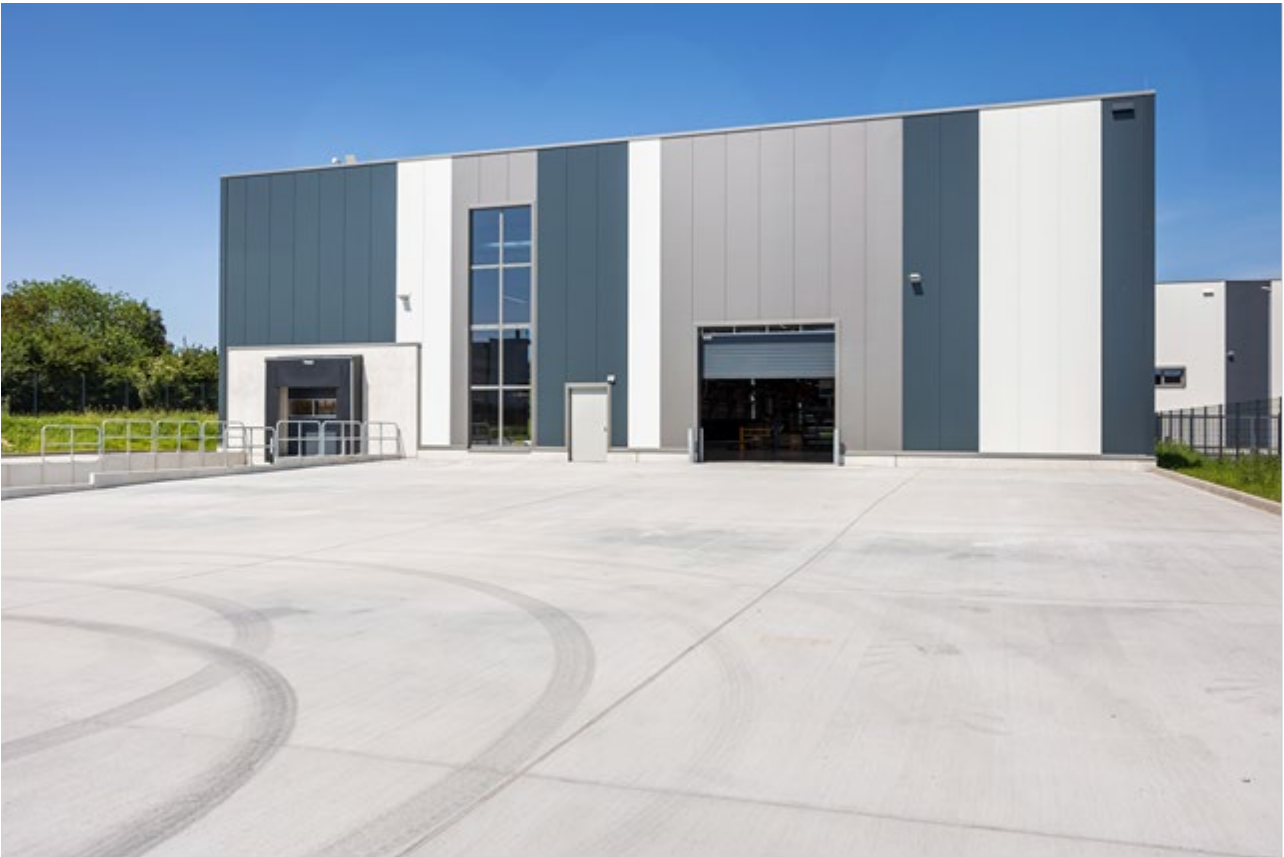
Exterior view of the new production hall, Credit: © GOLDBECK
