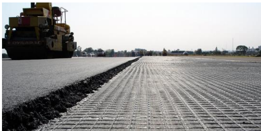
Fig. 3 HUESKER Asphalt Reinforcement_HaTelit: HaTelit® construction site photo
