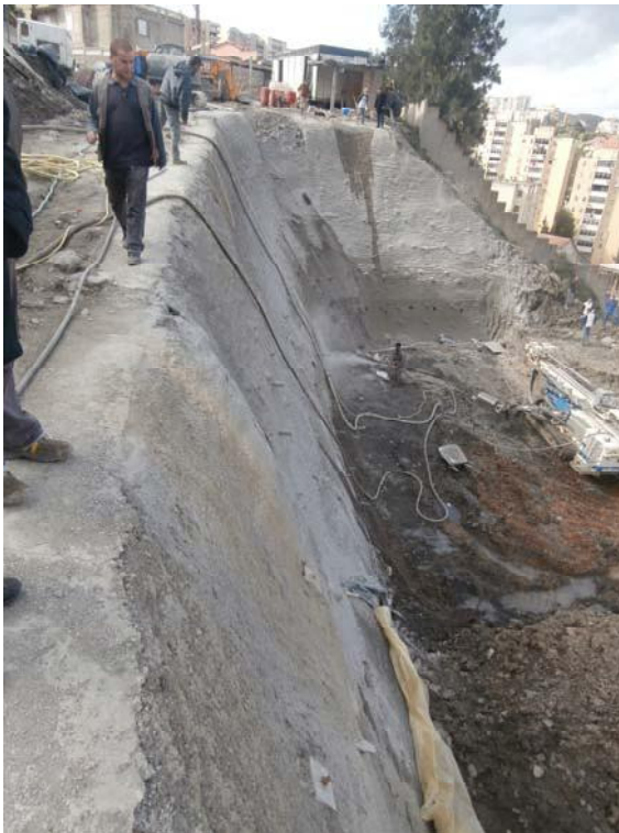
Figure 16. Anchorage and jet grouting of the excavated sliding surface and then implementation of a drainage géocomposite
