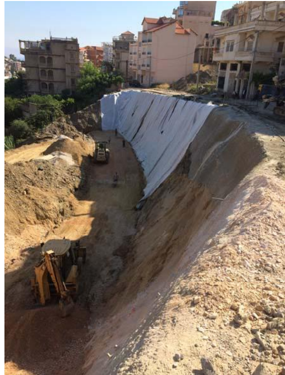
Figure 16. Anchorage and jet grouting of the excavated sliding surface and then implementation of a drainage géocomposite
