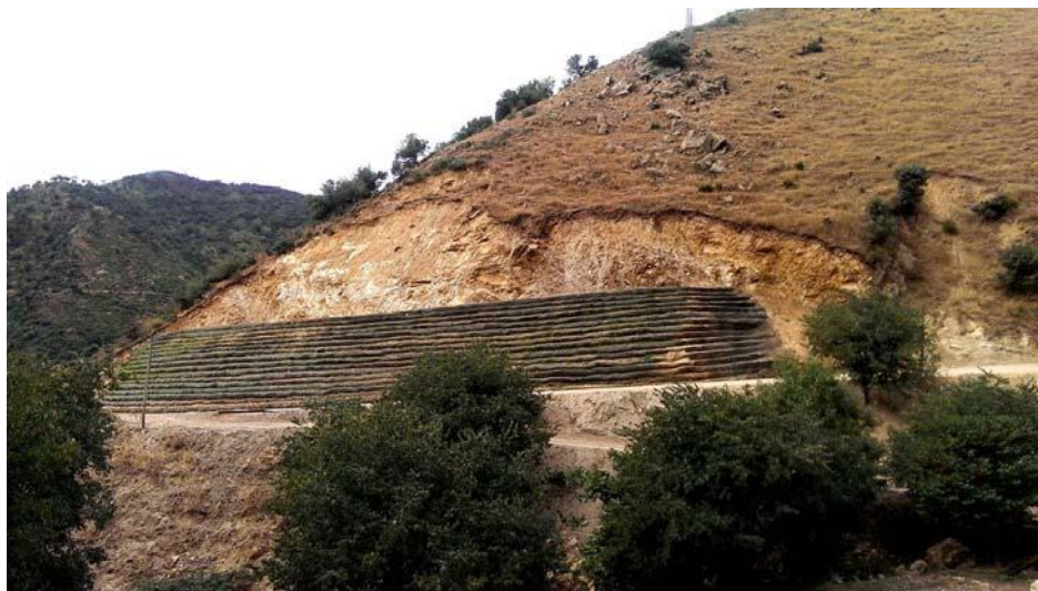
Figure 16. Earthworks completed – start of the greening of the facing
