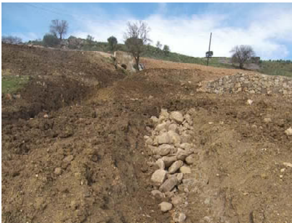
Figures 3 et 4. Examples of treatments with drainage trenches and spurs.
