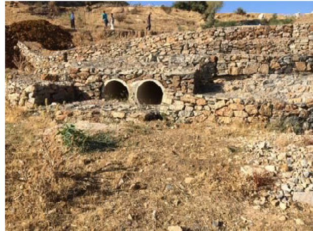
Figures 1 et 2. Examples of gabion toe
