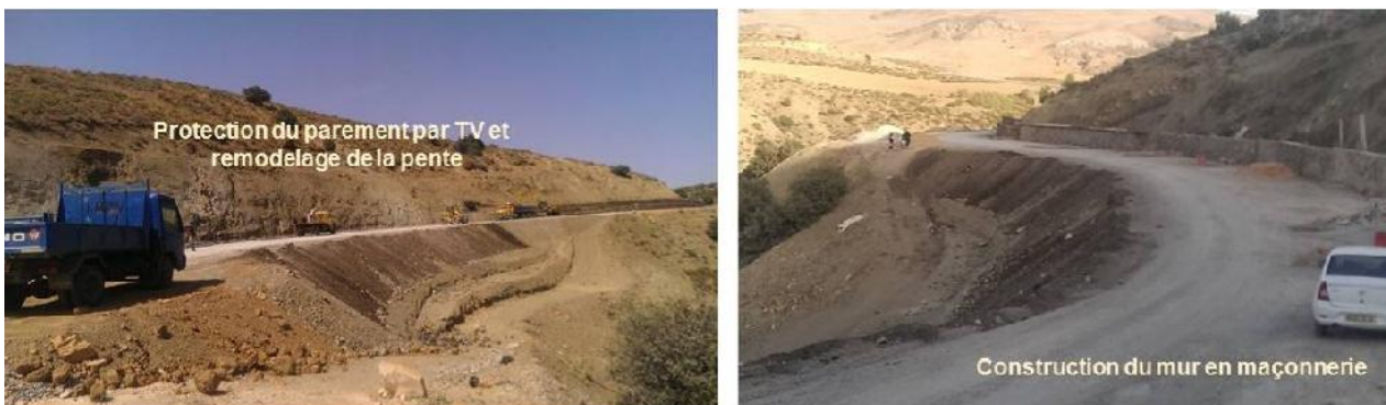
Figure 9. Building of the GRS
