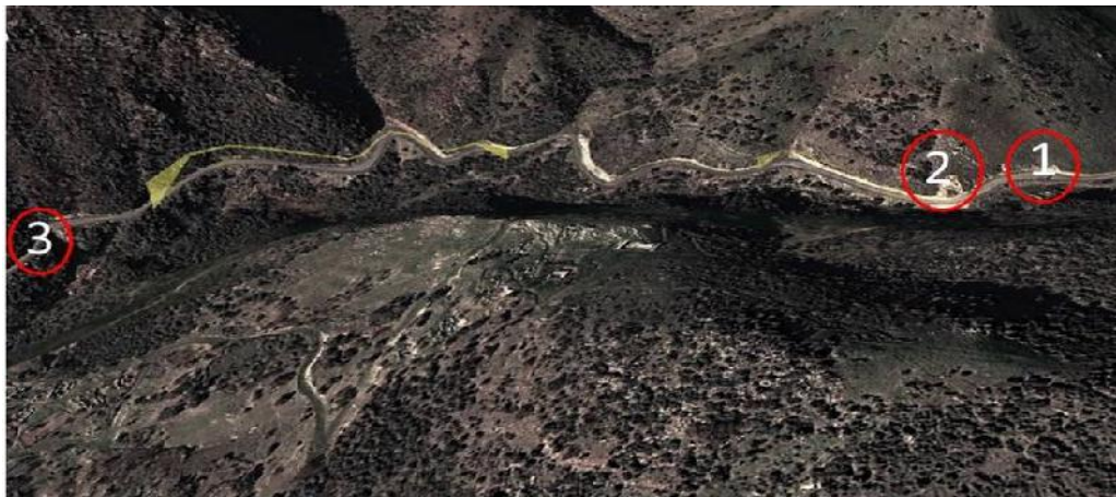
Figure 12. 3D View and position of the different slidings along the RN66 Road
