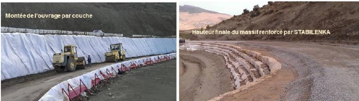
Figure 9. Building of the GRS
