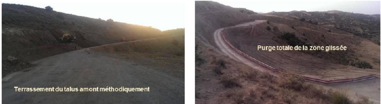
Figure 7. Widening of the road uphill and removal of the slid materials
