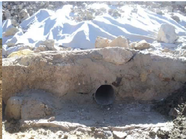
Figures 3 et 4. Examples of treatments with drainage trenches and spurs.
