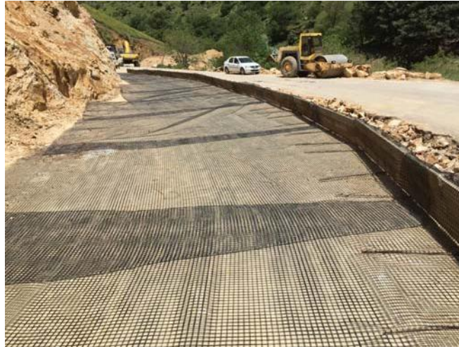
Figure 14. Construction of the reinforced slope with Fortrac Geogrid, layer by layer
