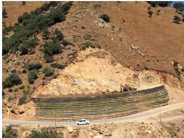
Figure 15. Construction of the reinforced slope with Fortrac Geogrid and compacted material
