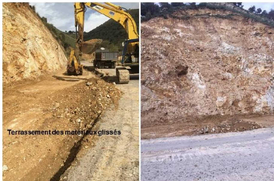
Figure 13. Removal of slided material and levelling
