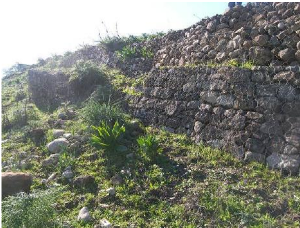
Figures 1 et 2. Examples of gabion toe
