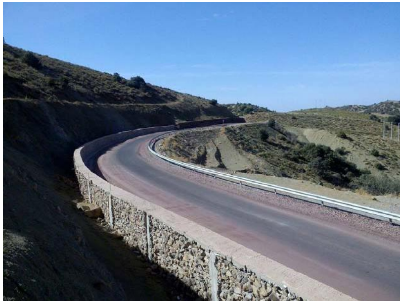
Figure 11. View of the finished project
